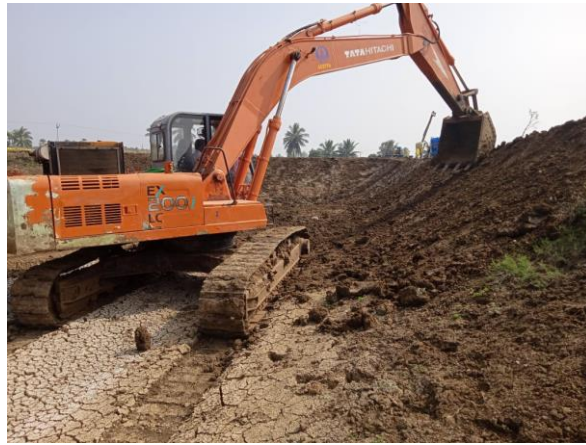
Fig 1: Pond construction work in Nagapattinam
